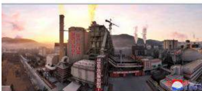
Sangwon Cement Complex Vows to Product Hundreds of Thousands of More Tons of Cement This Year | January 12, 2025
